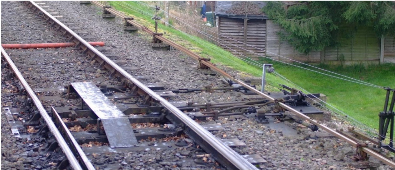
5 Facing point and detection at Bewdley, SVR
